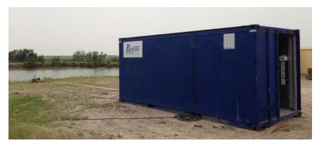
There is no pretreatment prior to the **Cuf** which eliminates the need for a clarifier and other pretreatment infrastructure. A small dosage of coagulant is added in-line where concentrated sweep floc occurs in the **Cuf** system. Coagulant dosage is less than the existing plant. No polymer or other process chemicals are added. The results of this pilot are consistent with other **Cuf** surface water pilot results.
