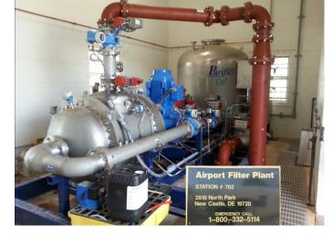
removed below the detection limit (<0.015 ppm) and slipstream of the Fe rich concentrate is less than 1% of flow. Filtrate is discharged directly to the clear well. Sustained flux is 825 GFD (1400 LMH) at a typical TMP of 12 psi (0.82 bar).
