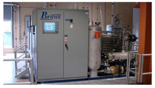
"The extracted groundwater is treated using advanced oxidation technology [Photo-Cat], which Lockheed Martin has found to be the most efficient, safe and cost effective way to treat site-specific chemicals of concern (CoCs), including trichloroethylene (TCE) and 1,4-dioxane." Lockheed Bulletin, 2011
