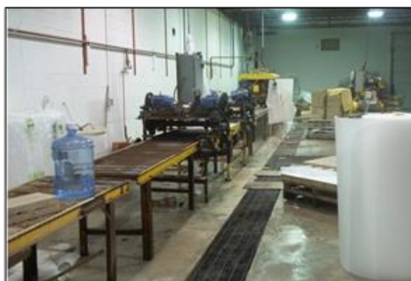
Beveling Line with Collection Trench and Water Distribution Line
